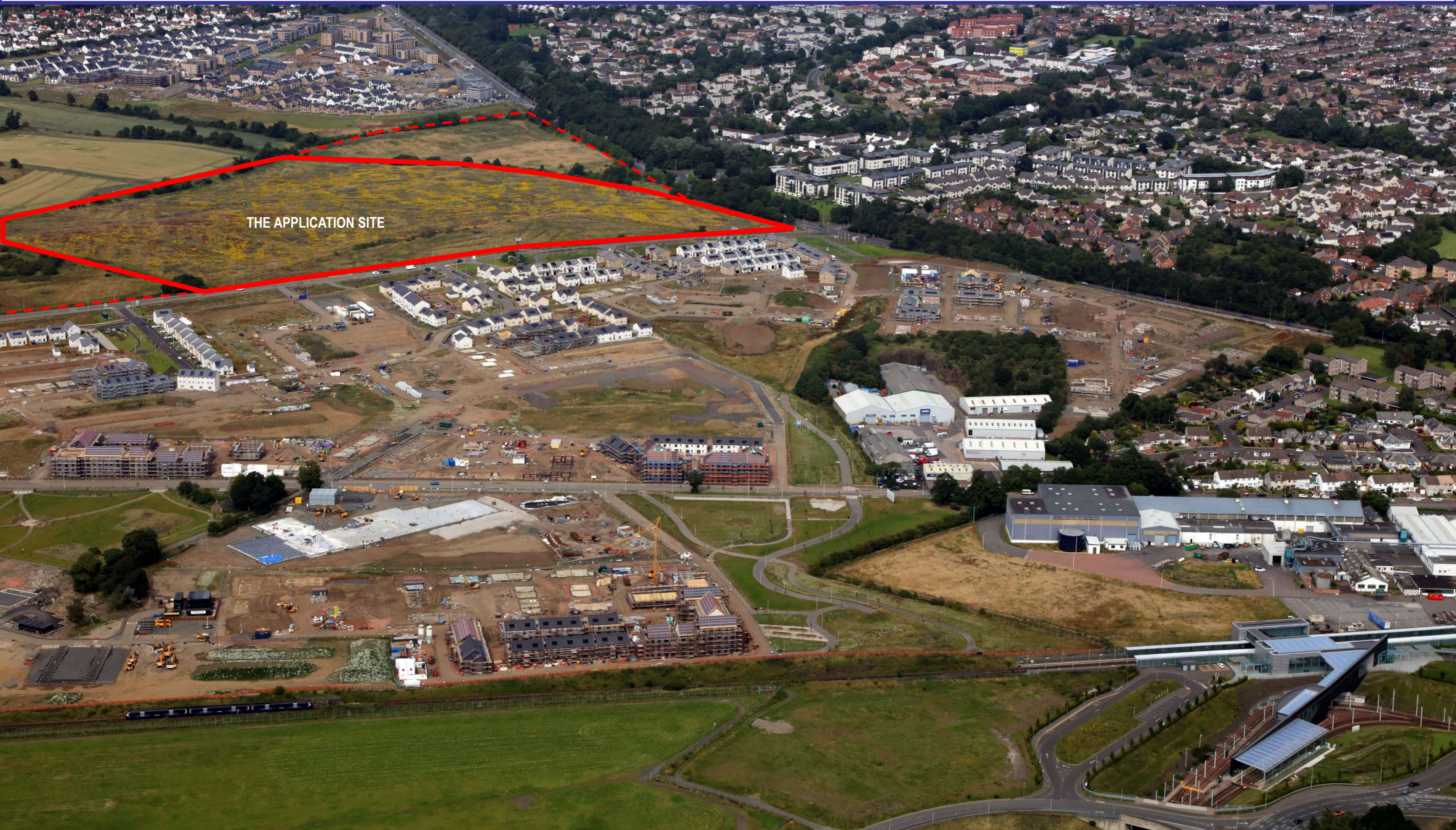
AERIAL PHOTOGRAPH FROM THE SOUTH
