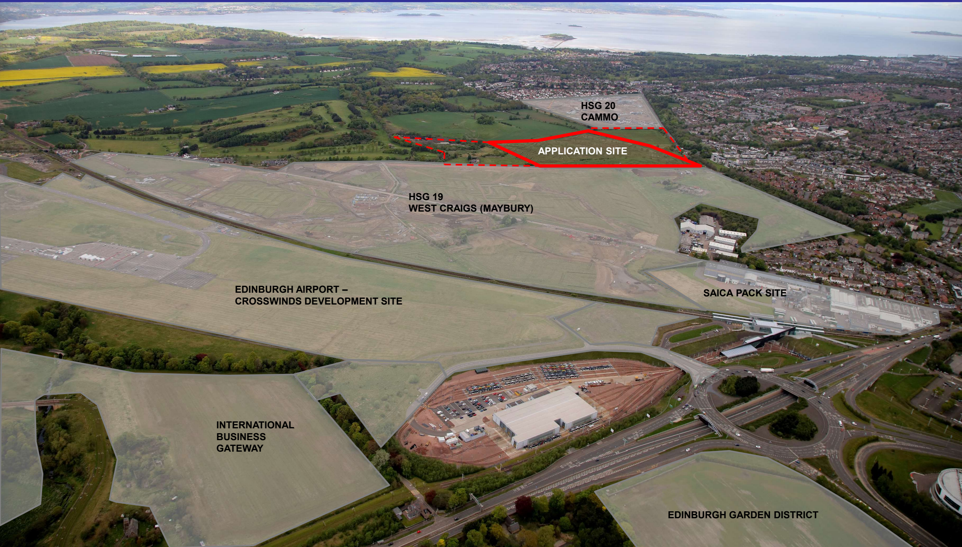
AERIAL PHOTOGRAPH SHOWING ONGOING AND FUTURE DEVELOPMENT OF ADJOINING LAND
